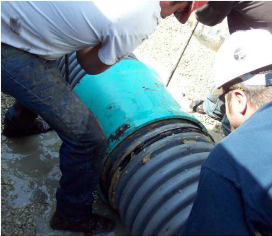
Figure 10.7: Slip Repair Coupling
